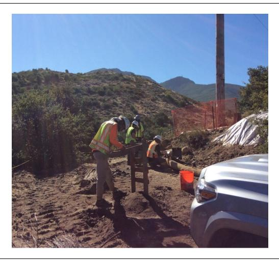
**Photo 3:** Cultural resources monitors were observed pre-digging and screening a ground rod trench along C 79B in accordance with the HPMP (MM CUL-1).
